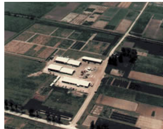
Figure 4. Elora Research Station
